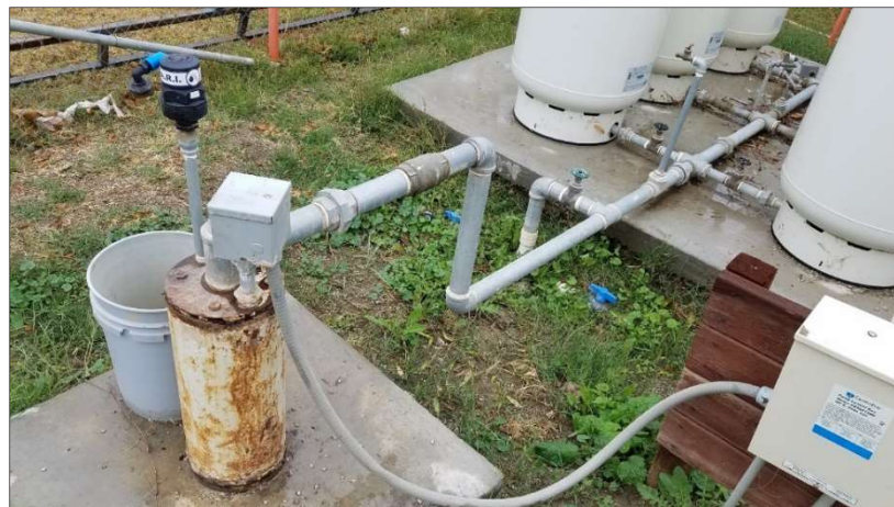
Manuela Garcia MHP existing well and above-ground piping
